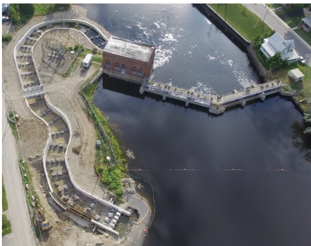
Nature-like fishway at Brookfield Renewable's Oswegatchie Project on the Oswegatchie River.
