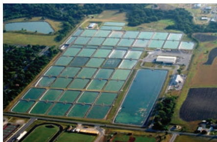
A.E. Wood in Texas was constructed in 1989 and illustrates a mid-century, large-scale fish production facility.
