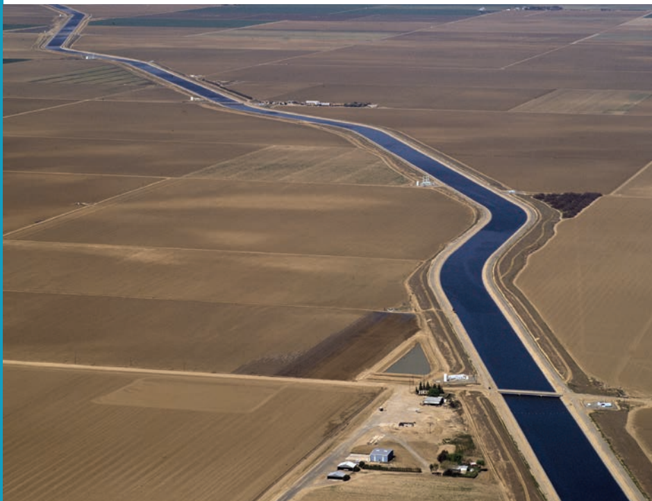
The California Aqueduct system was developed in the 1960s to store water and distribute it to 29 urban and agricultural water suppliers in Northern, Central and Southern California.
