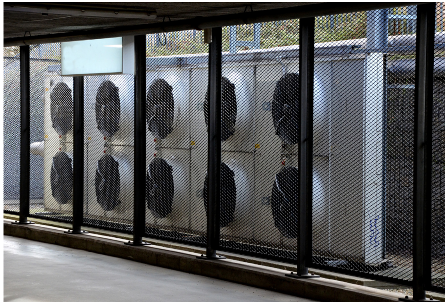
Heat pumps efficiently generate heat from an all-electric source, extracting heat and moving it where needed.
