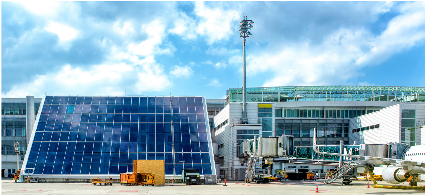
Solar panels at Munich Airport, which has set a goal of reaching carbon neutrality by 2030.
