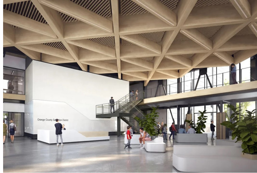
Mass timber with steel-braced frames support this roof for the Orange County Sanitation District headquarters.
