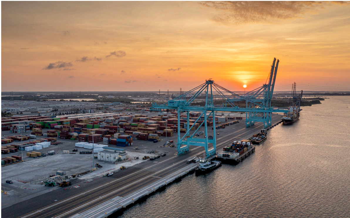
Bulkhead seawall at the Port of Jacksonville in Florida.
