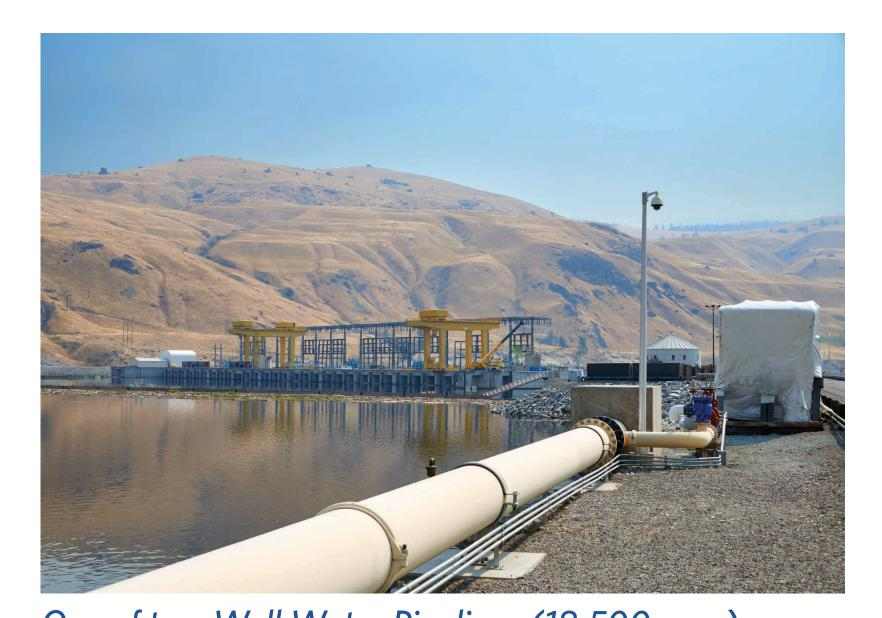
One of two Well Water Pipelines (18,500 gpm)
