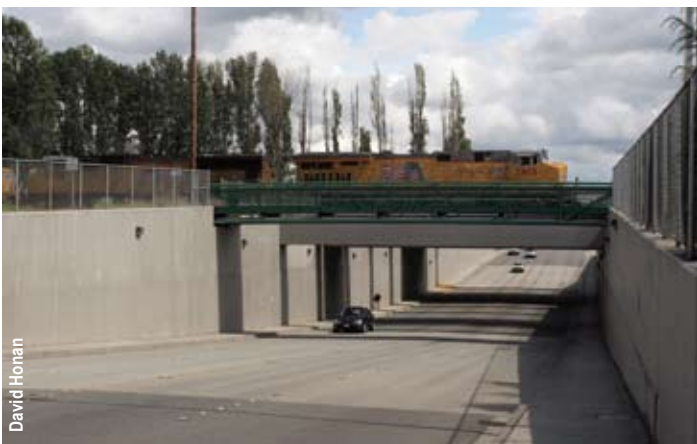
Grade-separated crossings make for safer motoring and can improve operational speeds for the railroads.
