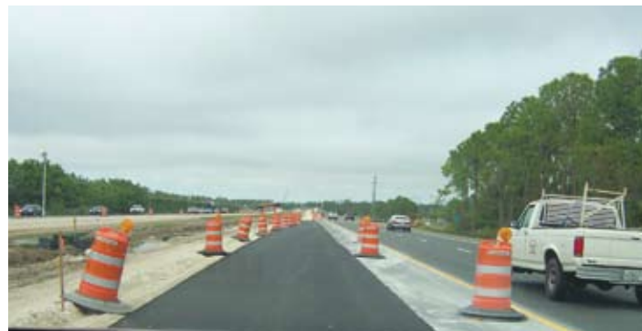
The new inside lane slopes the opposite direction of the outside lanes.
