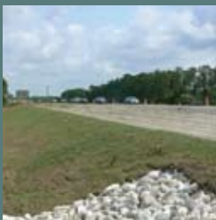
Stormwater, Environmental Work for I-75 pg. 9
