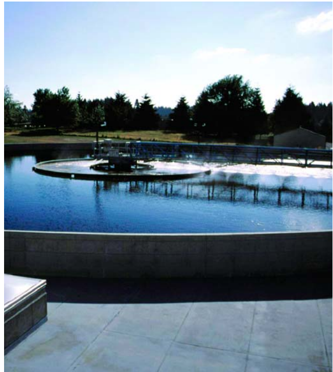
The evolution of the Durham Advanced Wastewater Treatment Facility involved continuous process improvements and optimization.
