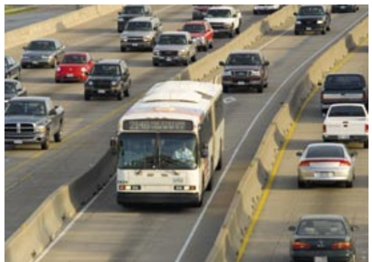
Houston's Northwest Freeway HOV lane. METRO operates 113 miles of reversible HOV lanes on five regional highways during peak hours to accommodate suburban commuters.
