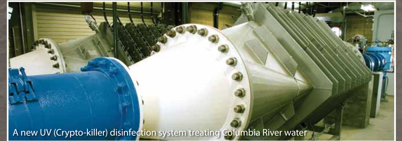
A new UV (Crypto-killer) disinfection system treating Columbia River water
