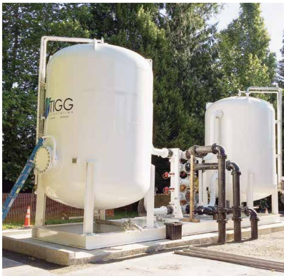
Granular activated carbon (GAC) treatment system for PFC removal, City of Issaquah, Washington
