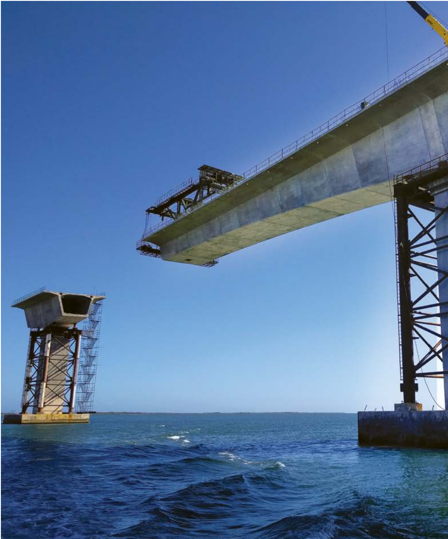
The massive structure includes nine 350-foot spans.
