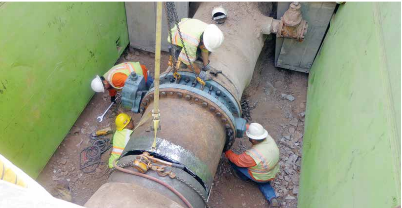
Inspection and condition assessment of a large diameter water transmission main.
