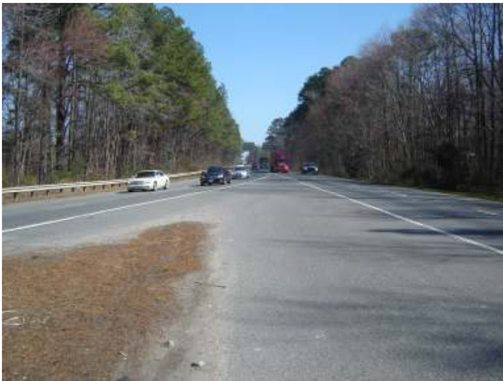
Photo 6 – U.S. 58 WB and U.S. 58 Business split; under alternative 1C (Flyover West), traffic exiting SPSA facility would be subject to unsafe merge conditions.
