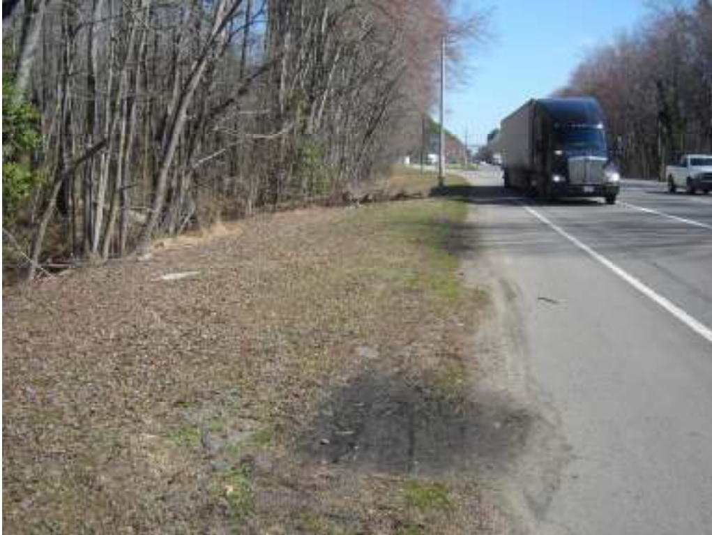
Photo 3- Merge to U.S. 58 EB from truck weigh station, which would create conflict and safety concern for Alternative 1A (Flyover East).
