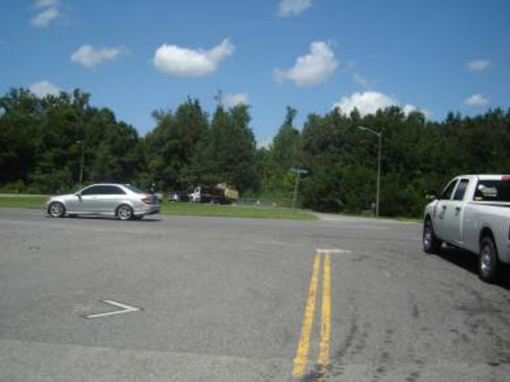
Photo 1 – Existing crossover from US 58 EB to Bob Foeller Drive, looking north, crossing US 58 WB.
