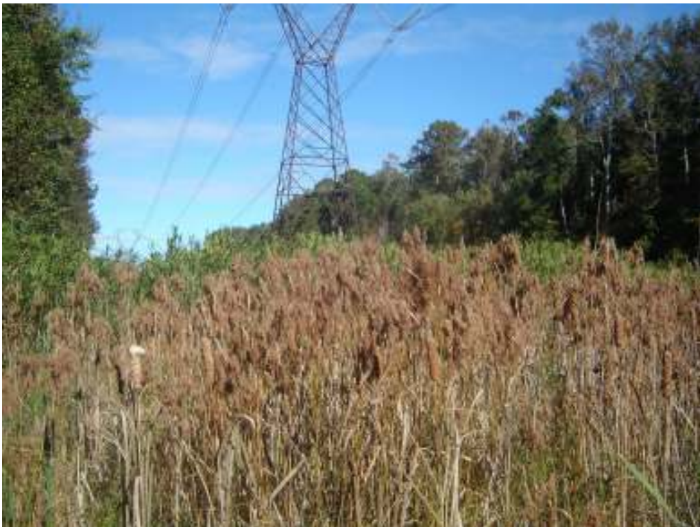
Photo 8 – Power line right-of-way containing emergent wetlands, seen from access path, looking north.
