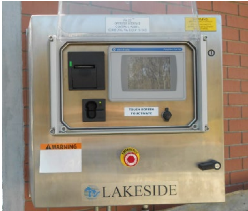
Figure 3-4. Lakeside RACS control station
