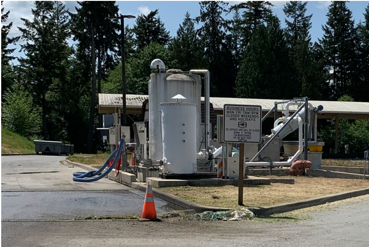
Figure 3-1. Existing septage-receiving station
