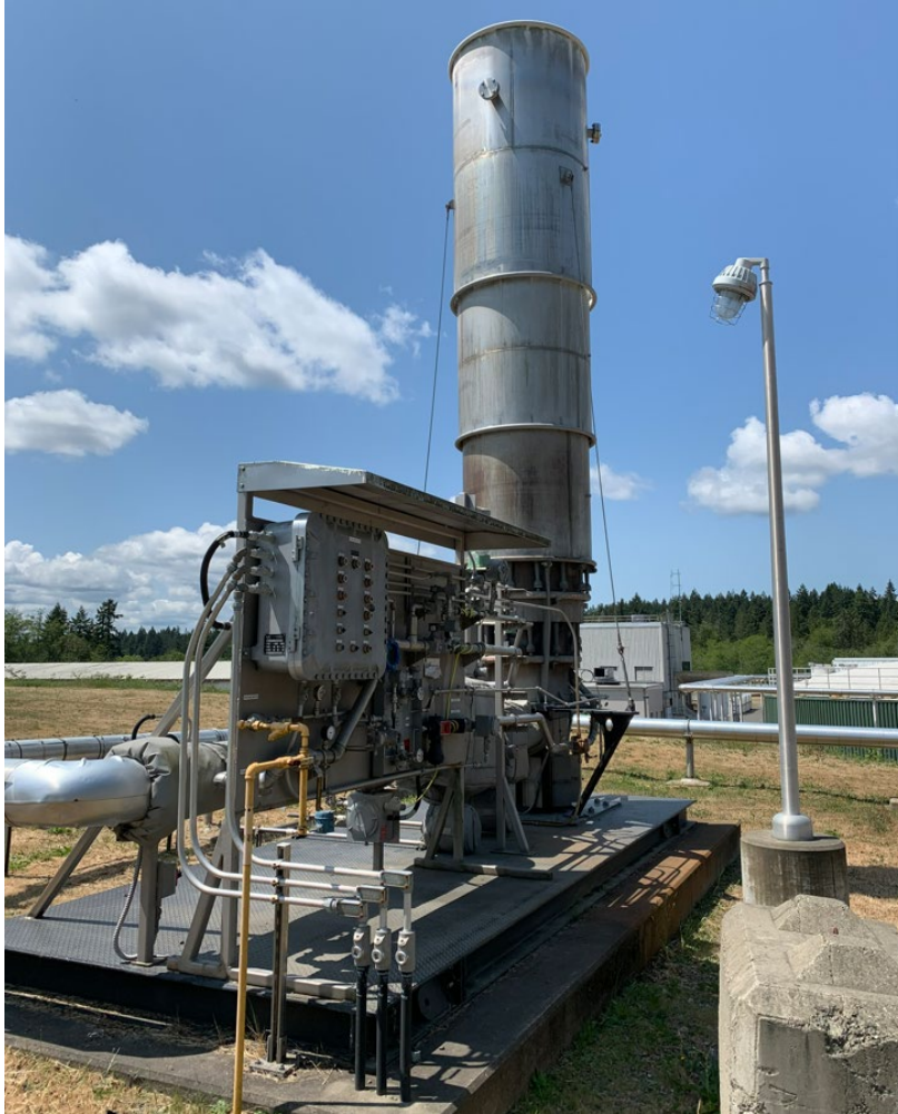
Figure 5-19. Existing waste gas burner with propane pilot (yellow piping in foreground) that will be updated to natural gas
