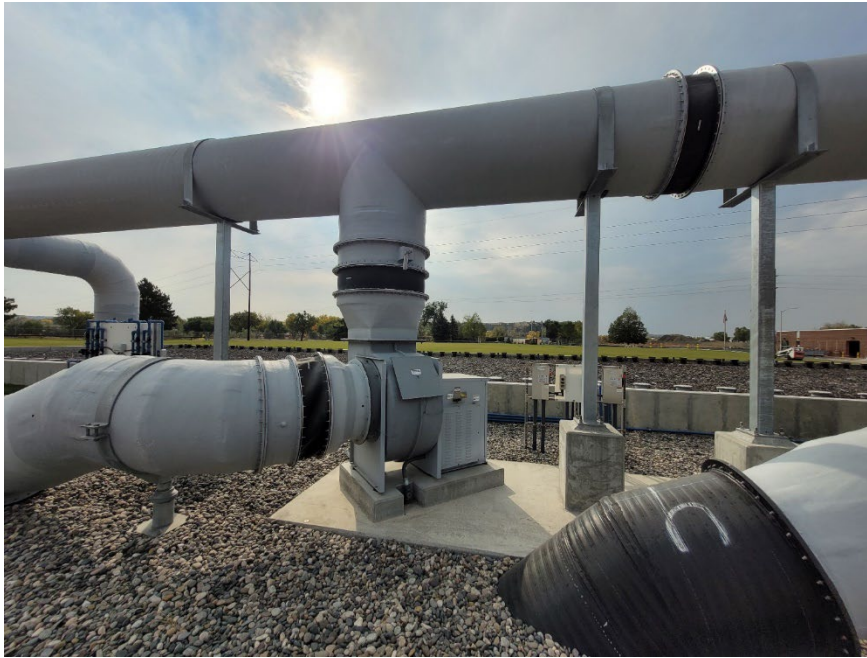
Figure 6-15. Foul-air duct (FRP and HDPE)
