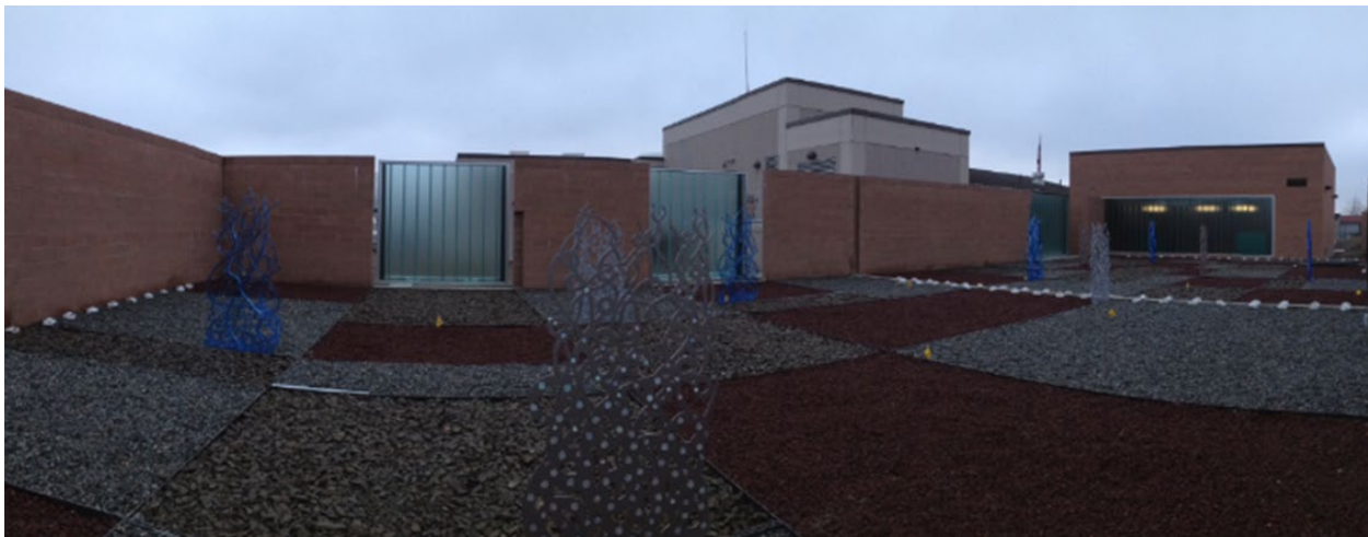
Figure 6-9. Bohn media biofilter, Wenatchee, Washington
