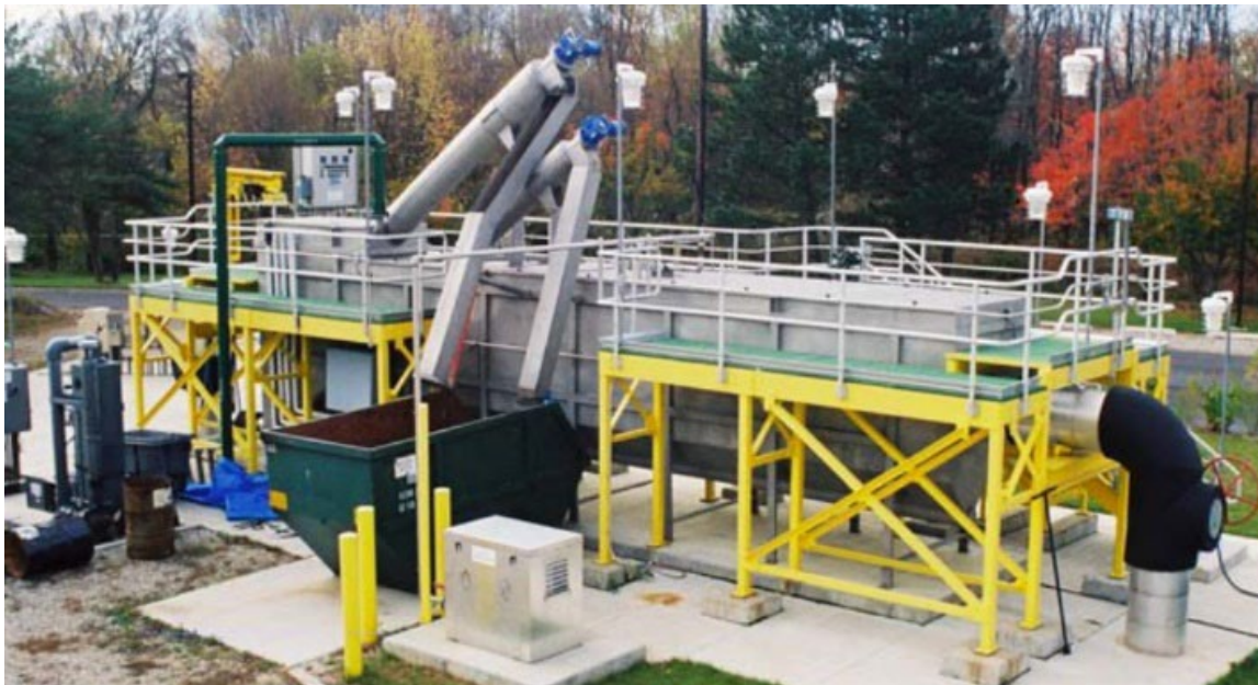
Figure 3-3. Example Lakeside Raptor Complete Septage Plant
