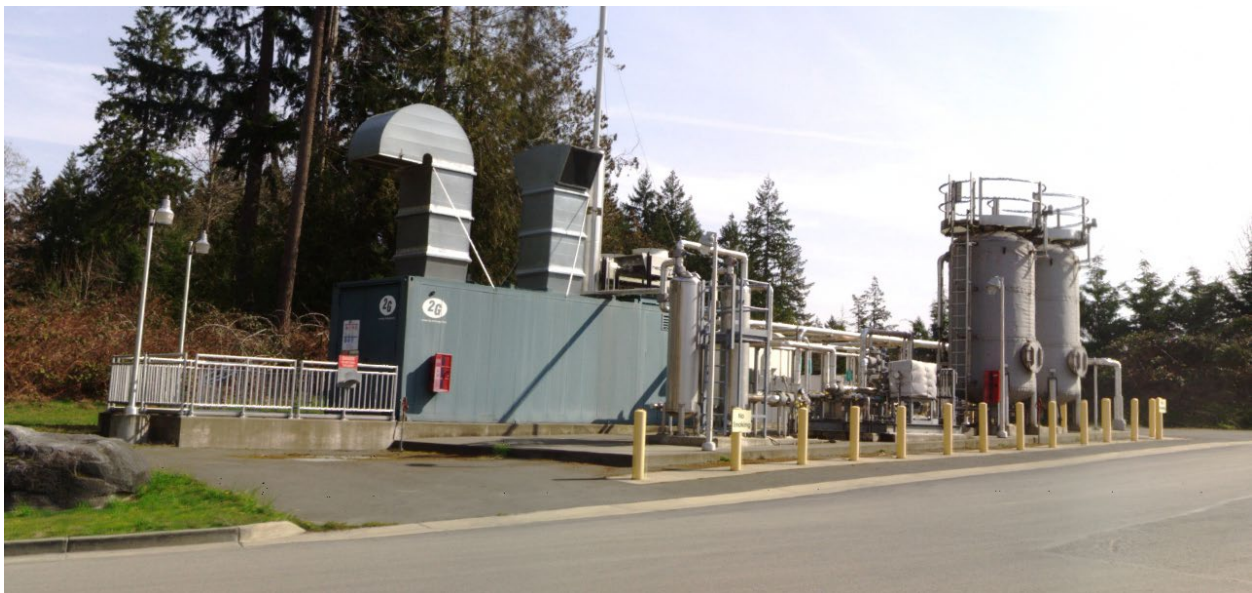
Figure 5-18. Existing CHP system with engine-generator and pretreatment \text{H}_2\text{S} and siloxane scrubbers
