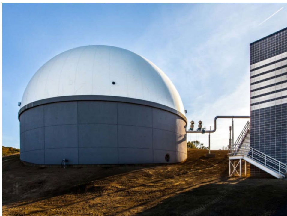
Figure 5-7. Example of gas-holding membrane cover
