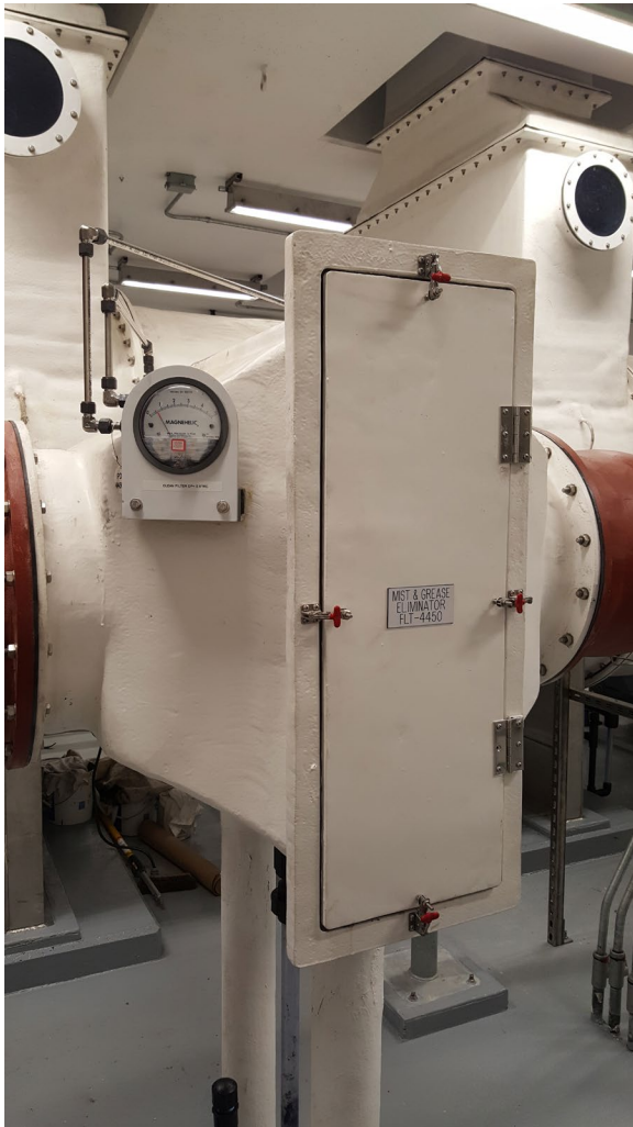
Figure 6-23. Grease filter with differential pressure gauge
