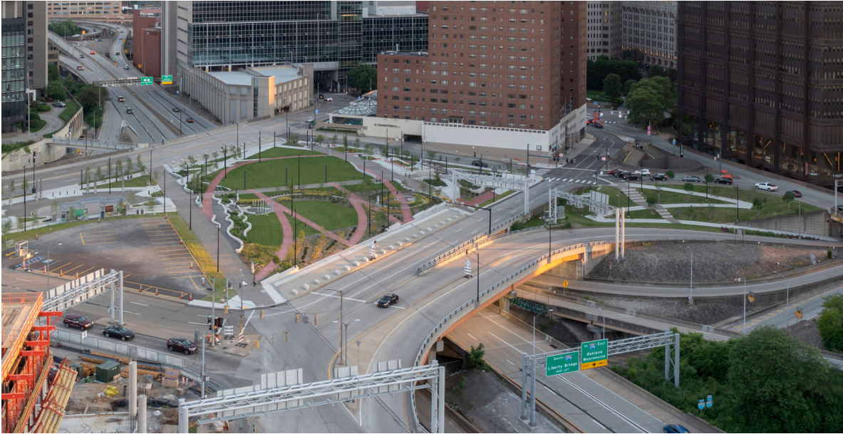
An urban park designed by HDR spans over a depressed section of I-579 in Pittsburgh.
