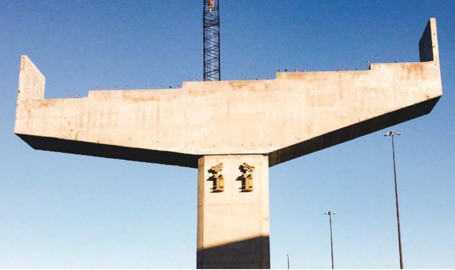
A hammerhead pier configuration was selected for pier locations where possible. Pier caps are 61 ft wide and 11 ft deep over the columns. The cast-in-place concrete caps are conventionally reinforced.
