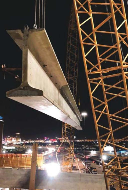
Installation of a California wide-flange (CAWF) girder at a straddle-bent location, with the neon lights of Las Vegas shining in the background. Compared with similar girder cross sections, the larger bottom flange of the CAWF shape allowed for more prestressing strands to be used.
