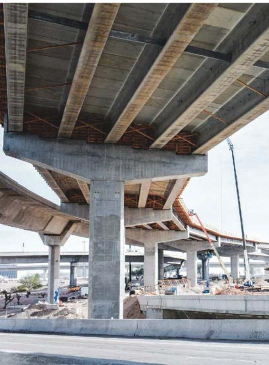
Chorded, precast, prestressed concrete girders provided an economical solution for Project Neon's high-occupancy vehicle connector bridge in Las Vegas, Nev. The temporary lateral girder bracing visible in the photo was removed when the structure was completed. All Photos and Figures: Kiewit Corporation.
