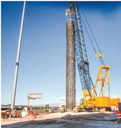
Installation of the reinforcement cage for a 11-ft 6-in.-diameter drilled shaft, located in the median of U.S. Route 95. Shafts were more than 100 ft deep in several locations.
