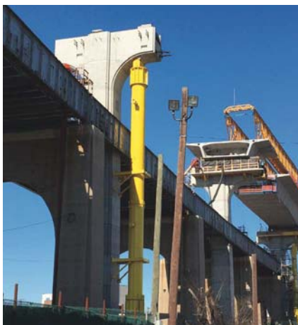
Temporary pipe strut bracing a northbound Type 1 pier.
