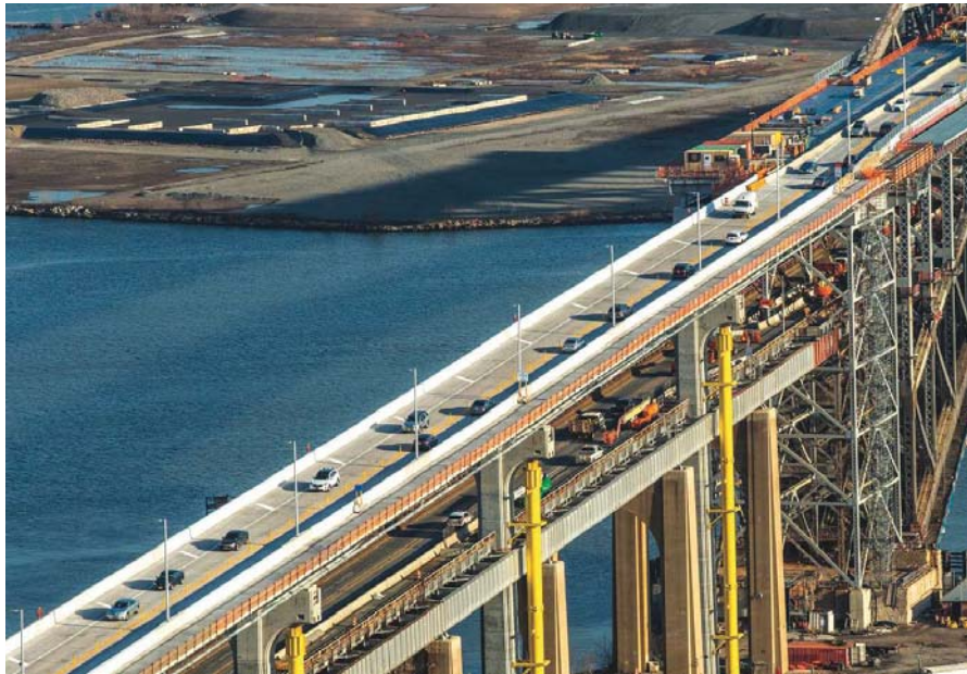
Traffic relocated to the new upper level of the Bayonne Bridge using the northbound approach structure. All Photos and Figures: HDR.
