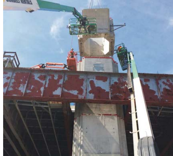
Erection of precast concrete column segment.
