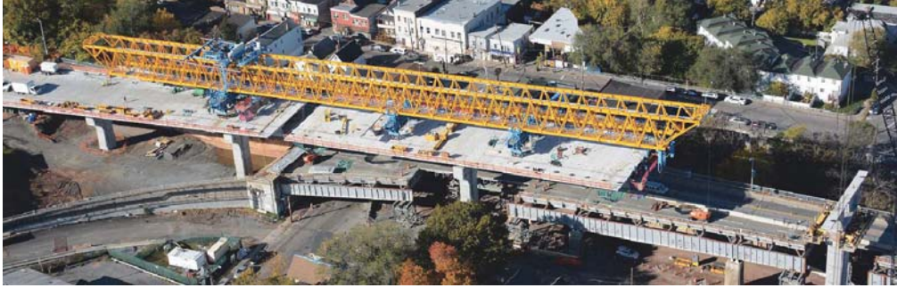
Balanced-cantilever construction for the Bayonne Bridge approaches.
