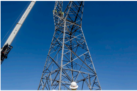
Transmission Lines PacifiCorp Gateway West
