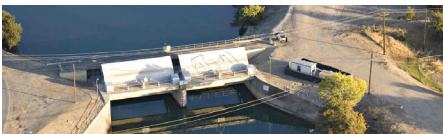
Delta Cross Channel Gates, Bureau of Reclamation, Sacramento, CA
