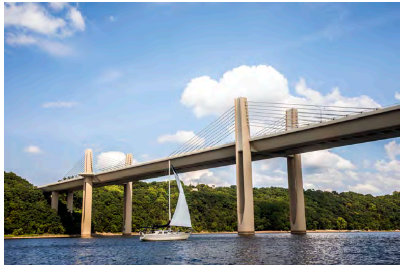
Designed to fit its environment, the St. Croix Crossing, built for the Minnesota and Wisconsin Departments of Transportation, uses an unusual extradosed design to reduce the number of pier supports. Other design choices included rounding corners to provide a streamlined look, subdued night lighting and an earth-tone color that helps blend with the surroundings.
