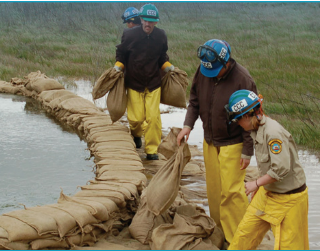
Above: Crew members place sandbags during flood fighting efforts (DWR).
