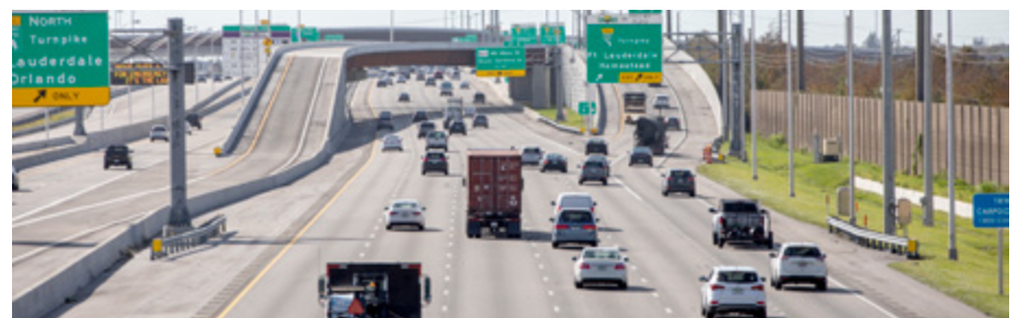
I-75 Express Lanes Project, Development and Environment (PD&E) Study, Broward County, FL
