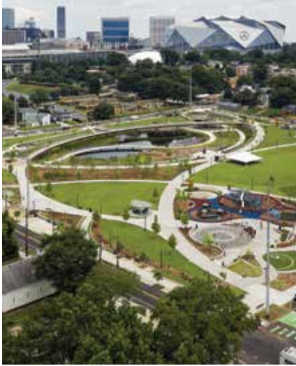
As an example of environmental justice considerations integrated into capital projects, the Rodney Cook Sr. Park in Atlanta has been designed to alleviate flooding by capturing and storing up to 10-million gallons of stormwater, while creating a vibrant community amenity to revitalize an underserved neighborhood in downtown Atlanta.
