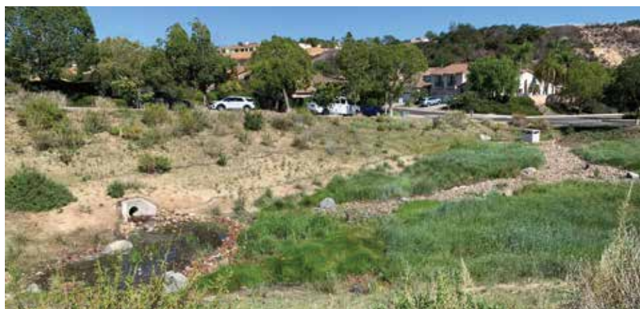
Ashley Falls Regional BMP provides total nitrogen, total phosphorus and total suspended solids control, as well as flow management in San Diego.
