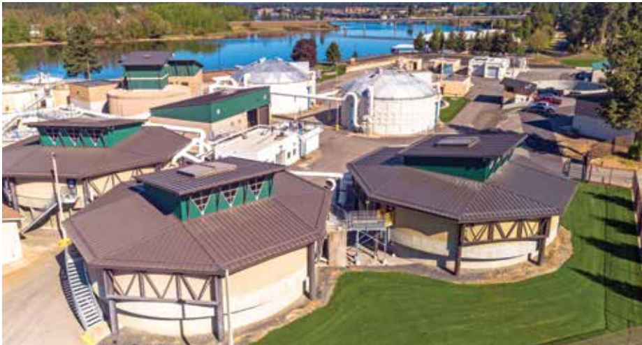
Advanced Wastewater Treatment Facility, City of Coeur D'Alene, Idaho.
